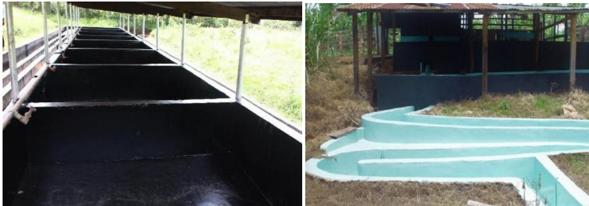
Figure 3.5: Well painted fermentation tanks and grading channel
