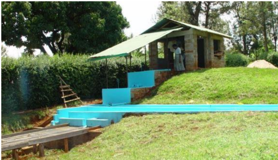
Figure 3.4: Small size pulping station
