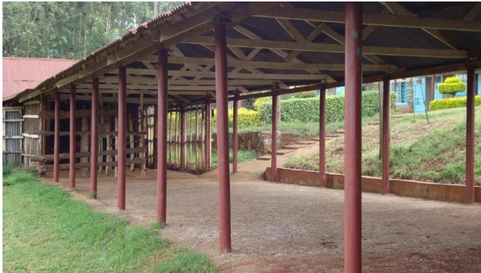
Figure 8.1: Well-maintained sorting shed
