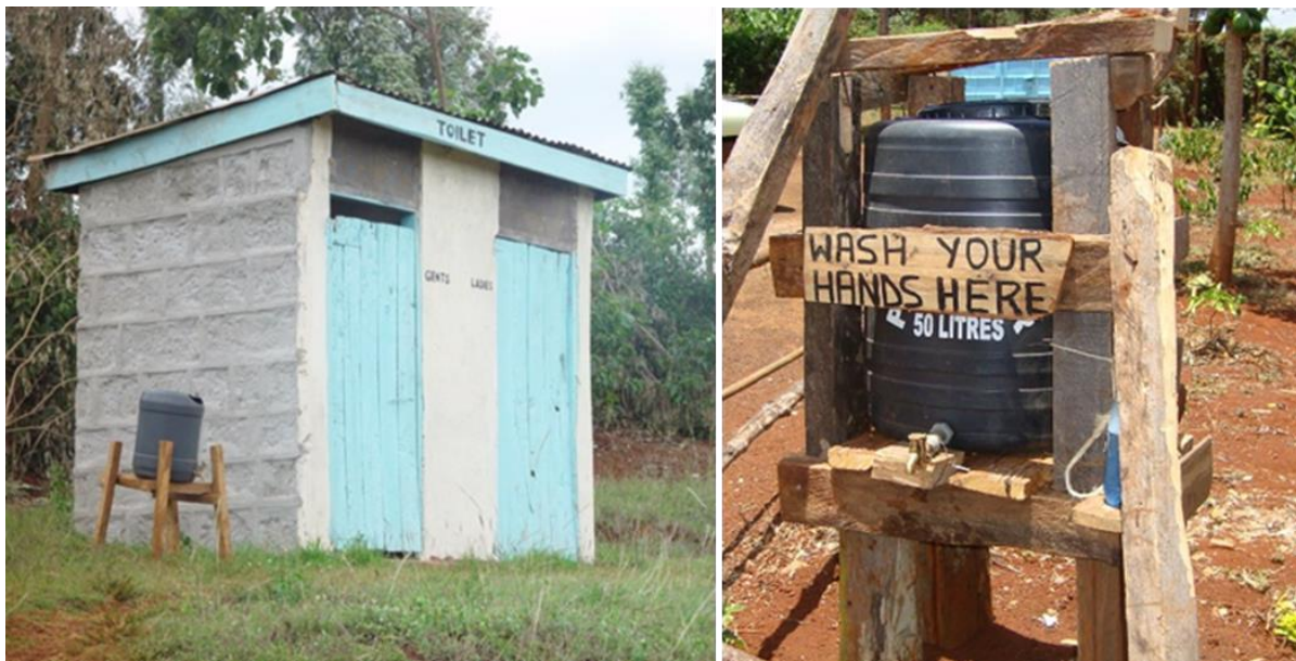
Figure 8.13: Well maintained toilet and with provision hand washing facility
